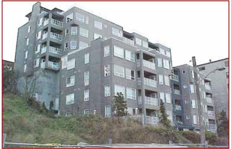
*Figure 2 – Energy-efficient walls that incorporate windows constructed with multi-layered, gas-filled, insulated glass with low-e films and thermally efficient window frames make it easy to justify an increased footprint and a higher window-to-wall ratio.*
