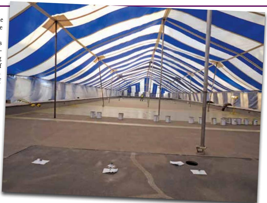
*A tent was set up over the entire pool area. The cold liquid-applied reinforced membrane system provides added protection over joints and cracks and around drains and other details. The solvent- and odor-free primer and resin system were important qualities during application.*
