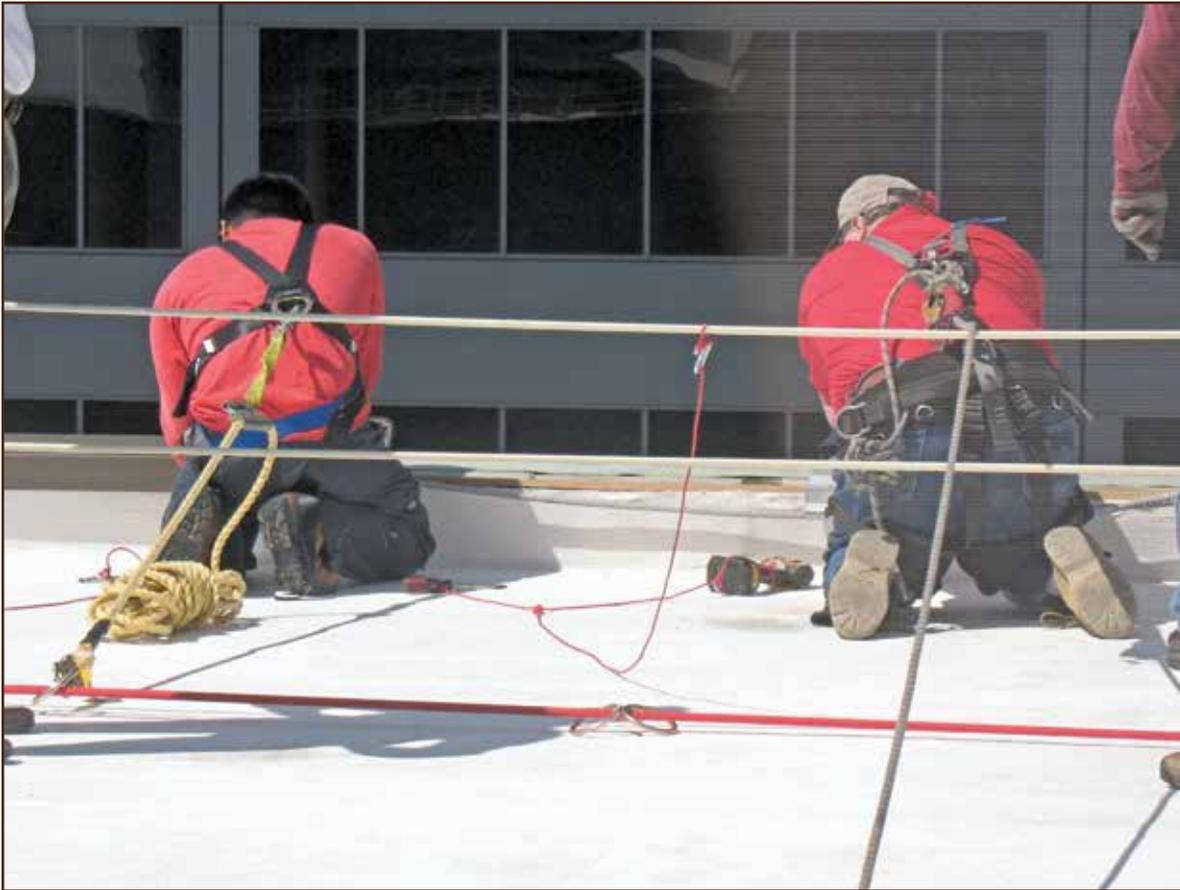
*Photo 4 – Workers employing fall restraint near a roof edge. Because the workers could possibly pass the edge, the systems were also designed for fall arrest.*
