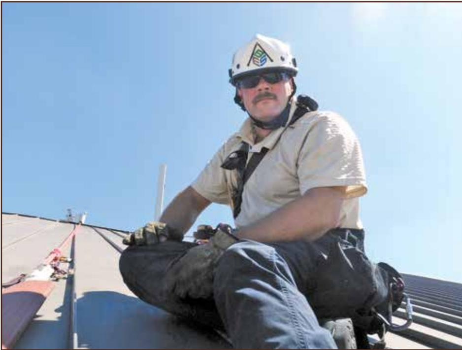
*Photo 2 – Technician near roof edge employing positioning (rope descender is positioned below right arm).*
