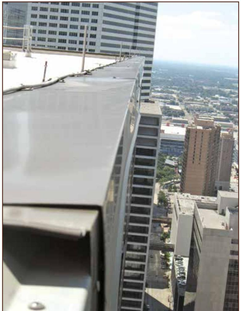
Photo 1 – Care must be exercised when employing fall restraint near roof edges.
