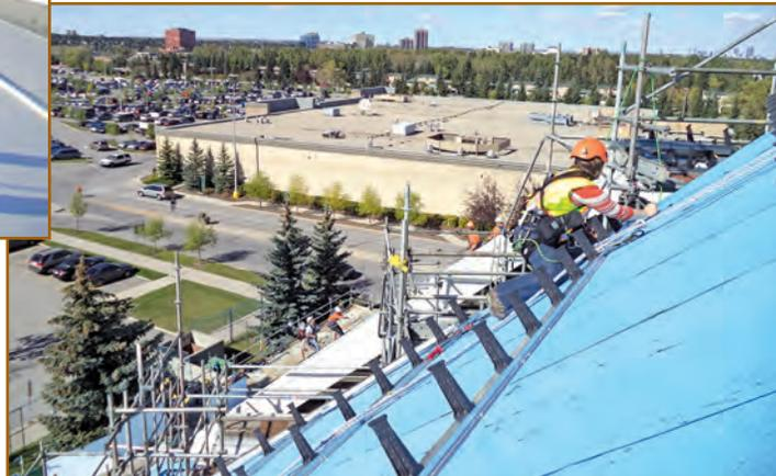
Technicians also rely on fall arrest devices, which act as backup safety devices and are used to stop a fall, slide, or uncontrolled descent. Any tools used during an investigation are attached to the technician at all times, allowing easy access to anything he or she may need. Technicians attach rope to structural roof anchors, either temporary or permanent; they can also tie off to structural members if necessary.
