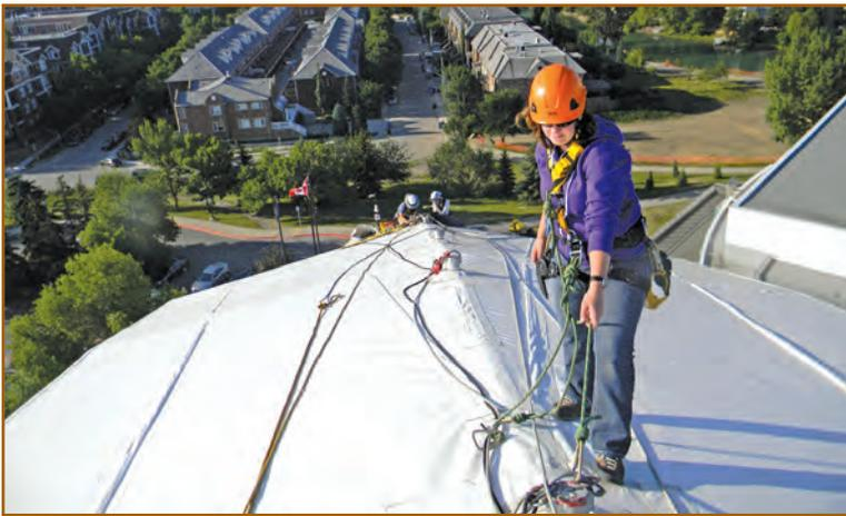
*Photo 4 - Mairead Walsh anchors her rope access equipment to a structural member of the Talisman Centre while conducting an investigation of the building's unique tent-like structure.*
